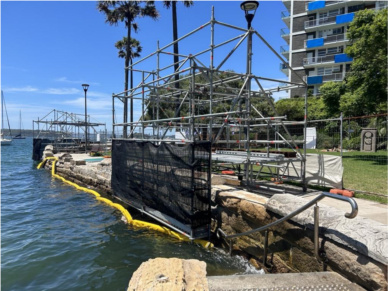
Beare Park seawall restoration using cantilevered scaffold to protect marine habitat. Image: City of Sydney
