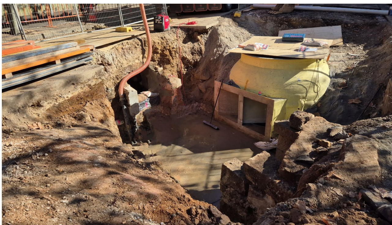
Image 7. New gross pollutant trap under construction, Broughton Street, Glebe. Photo by Adrian Smit / City of Sydney
